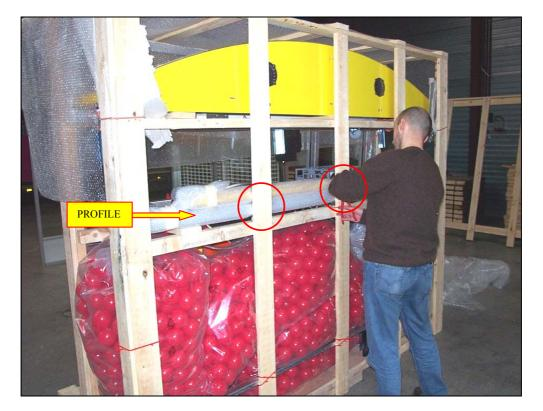
• Unwrap the longest pack and position the partitioning profile (= profile with 2x two pins) between the two sides (see drawing). Attach this profile in the provided holes with a rubber hammer.
